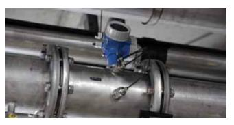
Ultrasonic measurement of biogas methane content and flow with the Prosonic Flow B 200
