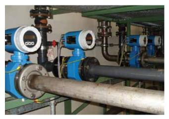
Reliable monitoring of flow rates with Promag electromagnetic flowmeter
