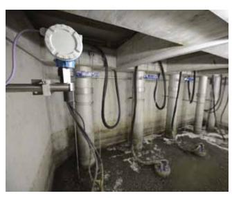
Dependable level measurement in the extensive sewerage system
